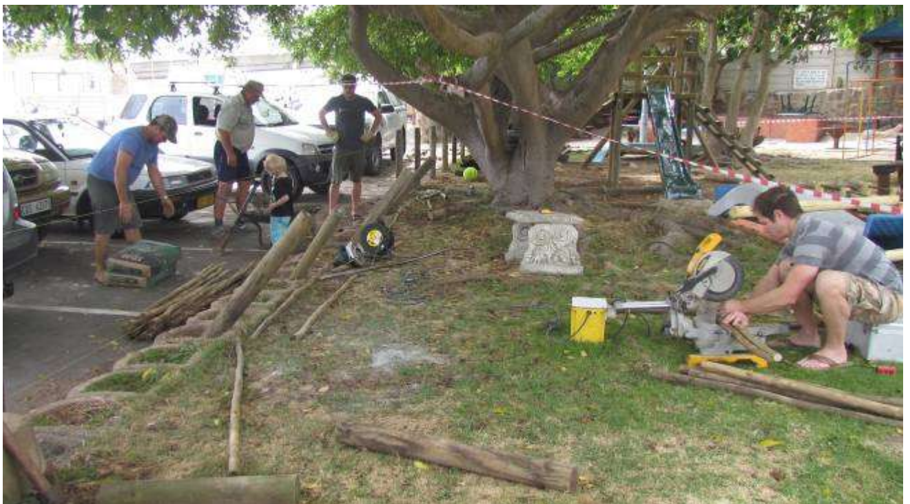
Edrich MvDonald, Geoff Keet, Geoff Scrembrucker and Greg Fenn busy erecting the fencing.
